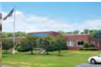
US Tsubaki Holyoke Plant
