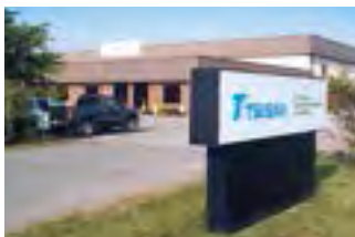
US Tsubaki Portland Plant
